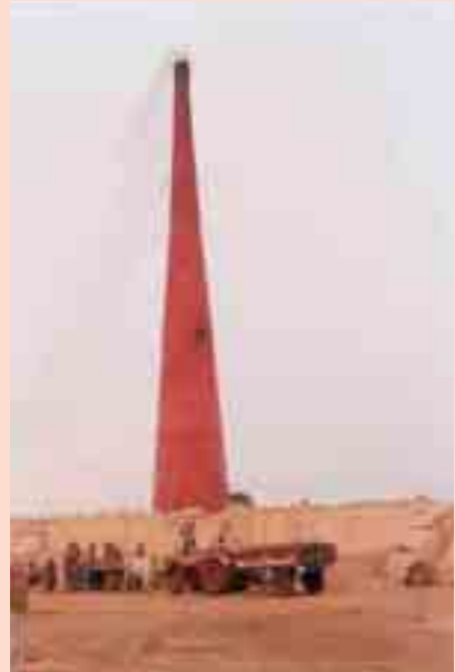
Figure 2 Fixed chimney BTK
