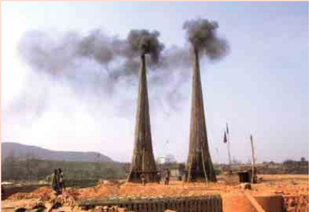
Figure 3 Moving chimney BTK
