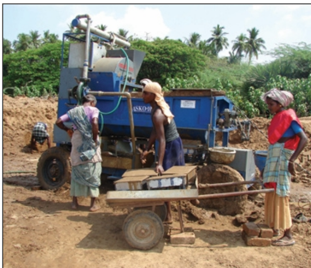
Reducing drudgery: Moulding machine for making bricks
