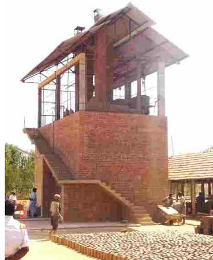
TERI introduced VSBK (Vertical Shaft Brick Kiln) in Kolar/Malur during 2005, which are more energy efficient and environment friendly (figure 12). The specific energy consumption of VSBK was the lowest among other types of brick kilns (figure 13).
