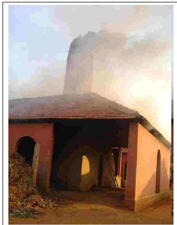
**Figure 4** Stack emission from a downdraught kiln
